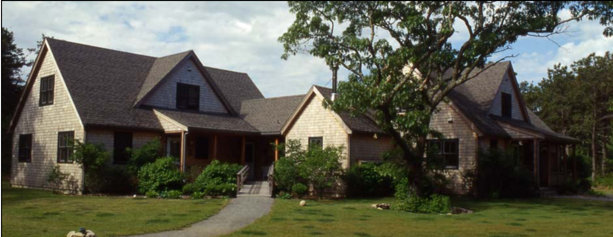
Affordable rental housing at Sepiessa Point (Regional Housing Authority photo)
