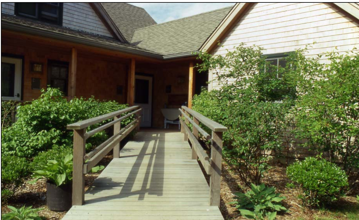
Affordable rental housing at Sepiessa Point (Regional Housing Authority photo)
