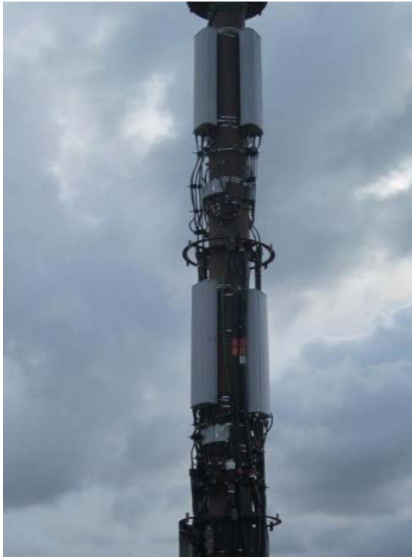
Figure 5: CMP without Covering
