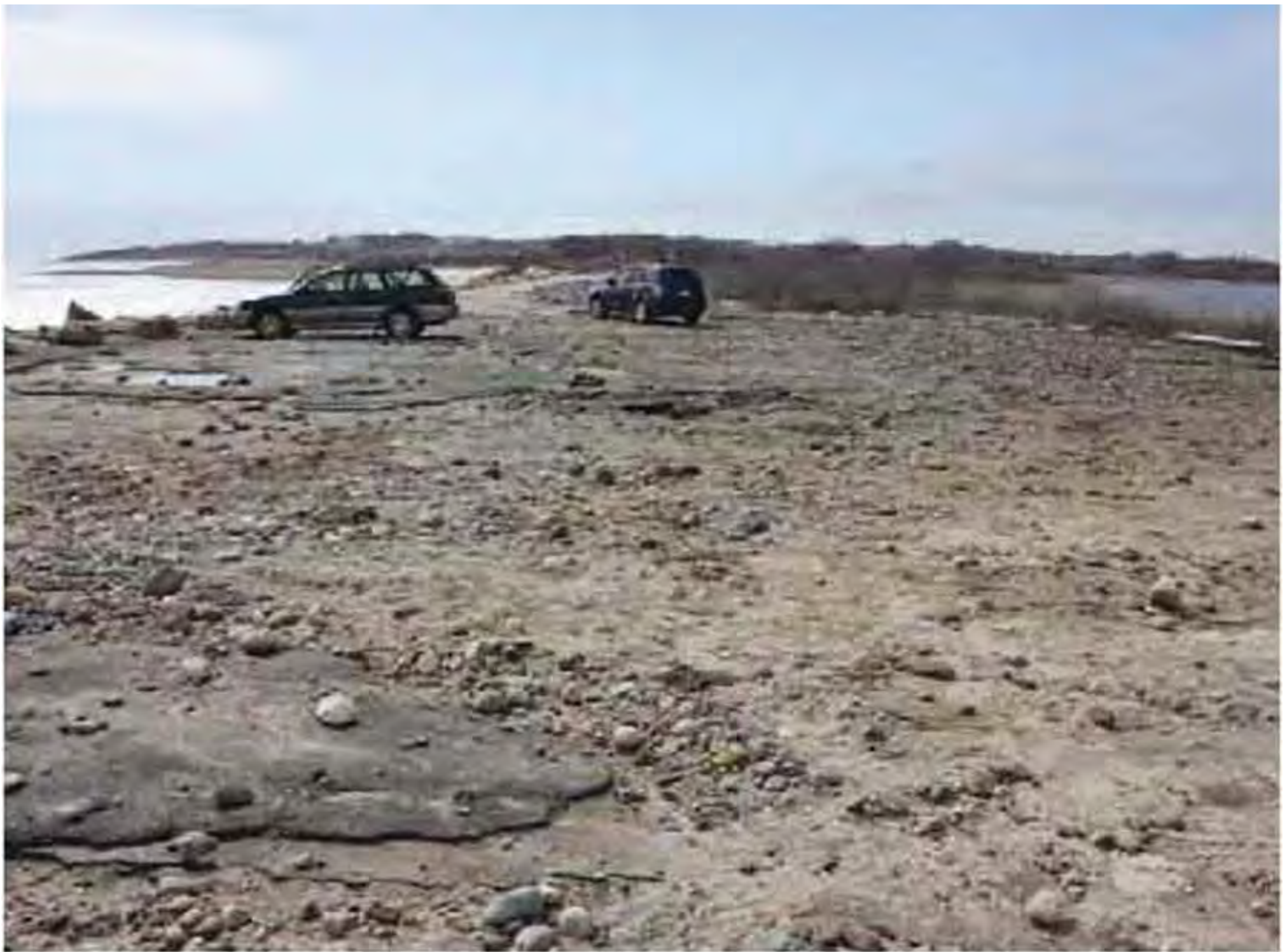
6 – Parking lot debris and damage following a severe storm event
