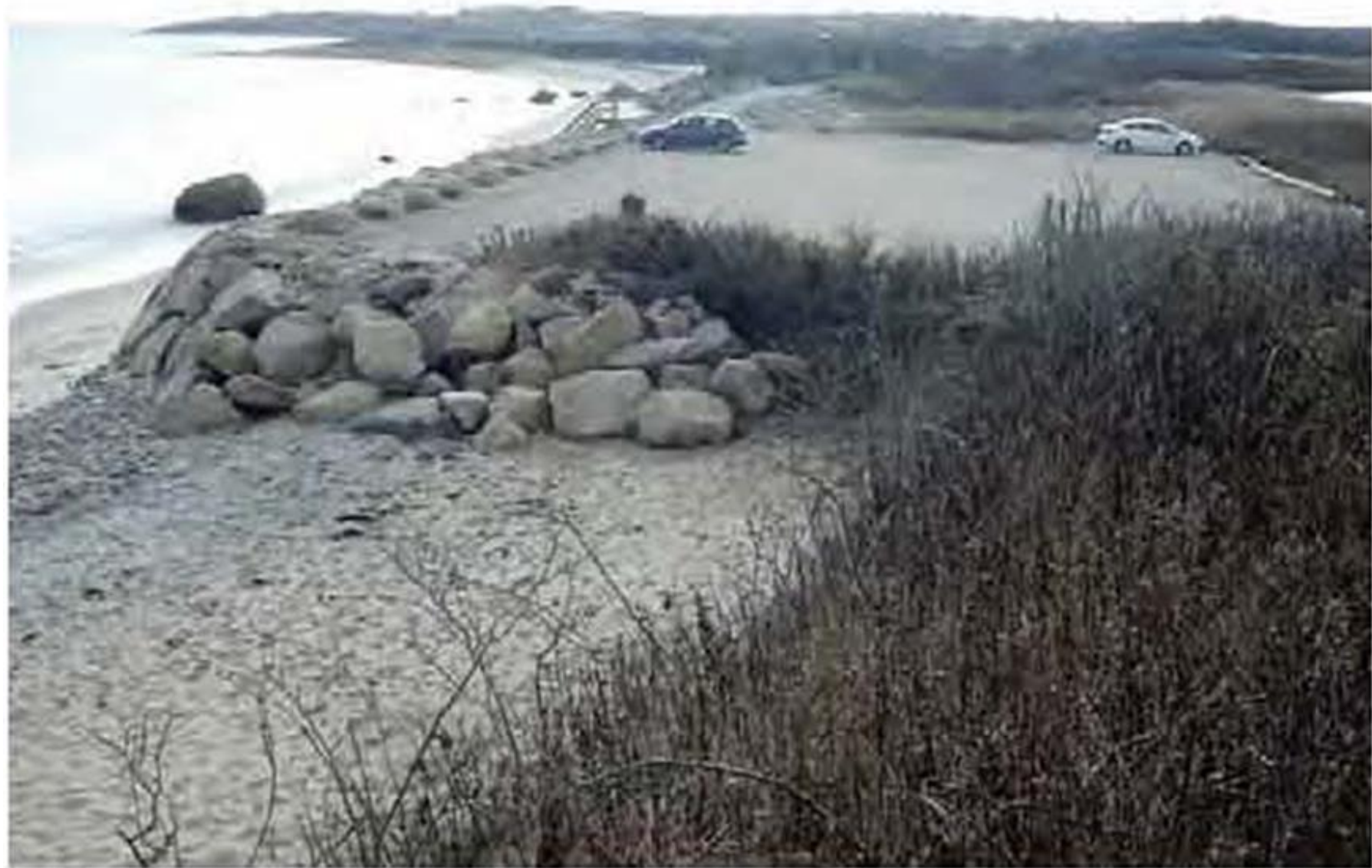
1 – Looking south to southeast across the Existing Town Lot
