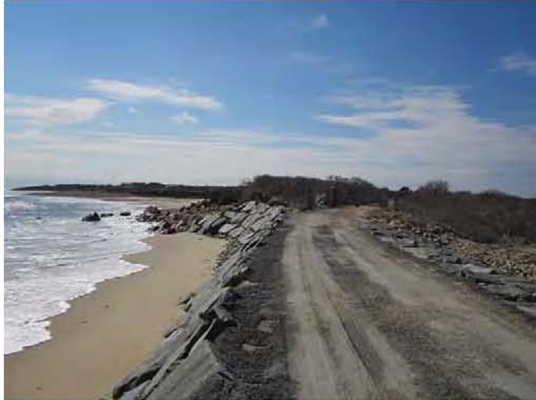
4 - Looking south to southeast along the existing Causeway Revetment
