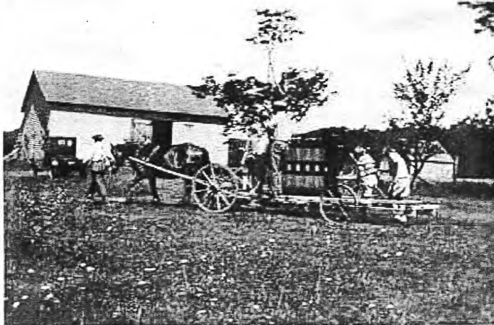
Figure 1 Cowbarn, 1920s, east elevation prior to conversion to residence (photo courtesy Polly Hill Arboretum).
