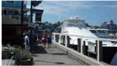
Figure 26 – Approximate scale of a permanent glass flood barrier at elevation 9.7 feet NAVD88
