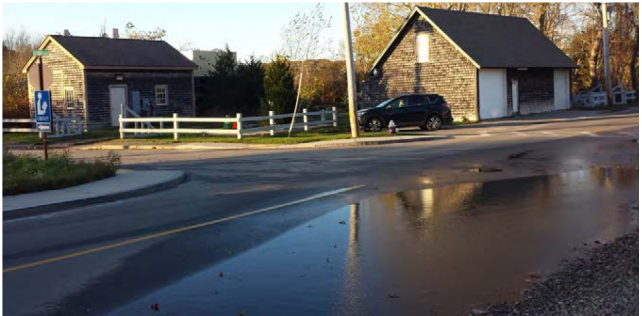
Above: Town sewer pumps at Dukes County Ave and School St are in a low-lying area vulnerable to flooding.
