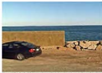
Figure 39 - End of Existing Seawall at Seaview Ave. at Farm Pond
