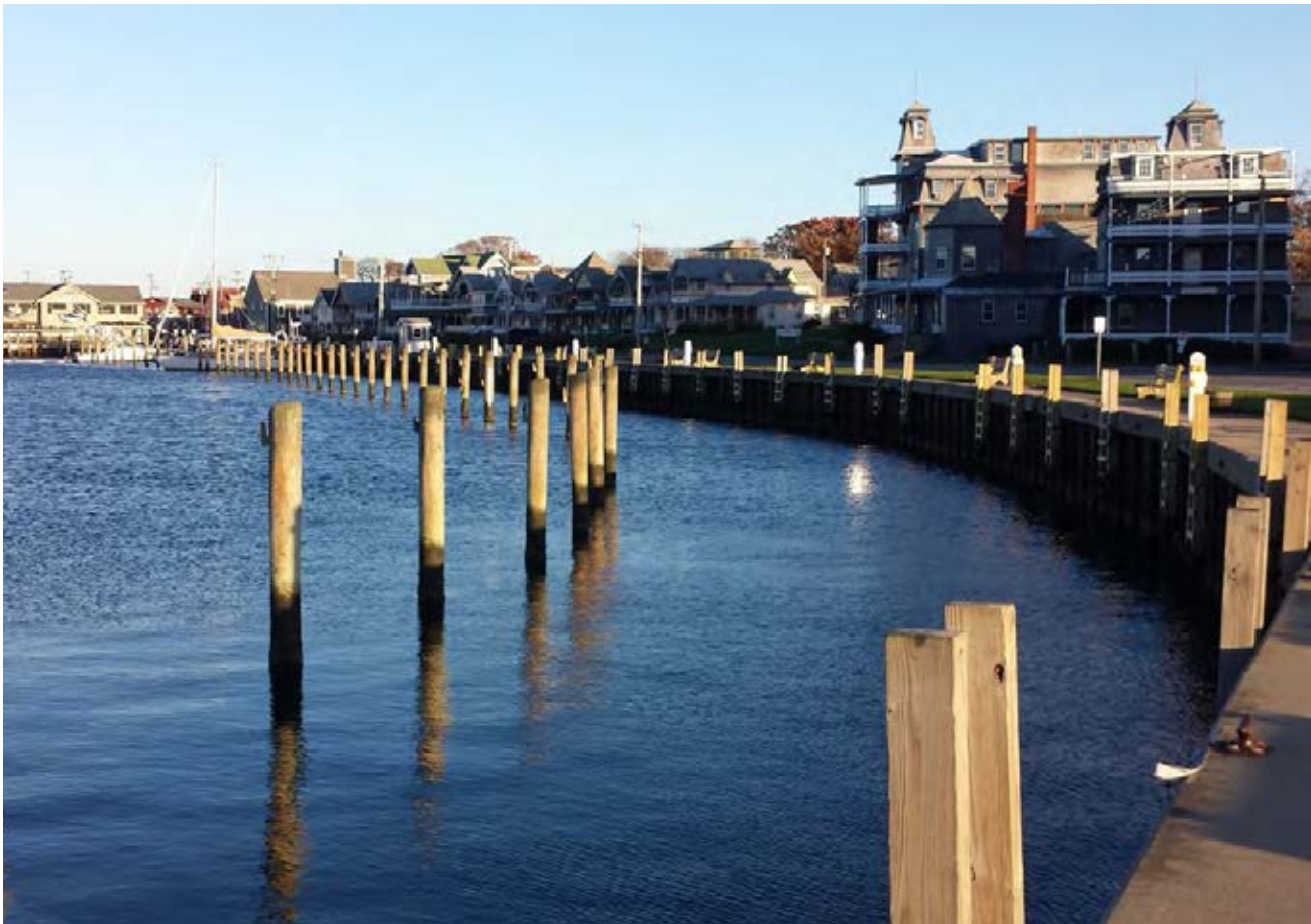
Lake Ave along Oak Bluffs Harbor is an important link through Oak Bluffs' town center. Its vulnerability to storm surge inundation will increase with sea level rise.
