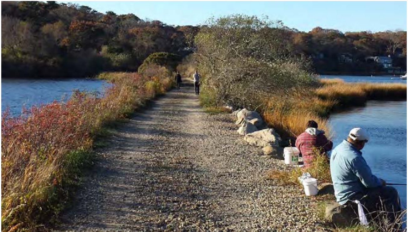
The causeway between Upper Lagoon Pond and Lower Lagoon Pond preserves Upper Lagoon Pond's freshwater environment from saltwater intrusion. Sea level rise could likely lead to high tides overtopping the causeway if it remains at its current elevation, which would wipe out this important freshwater habitat.
