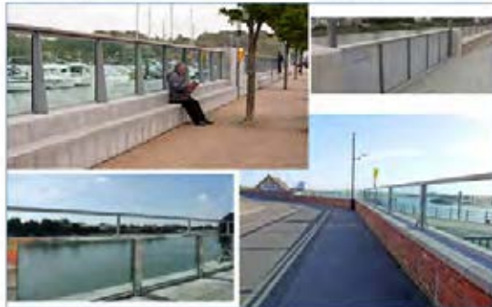
Figure 25 – Example photos of permanent glass flood barriers
