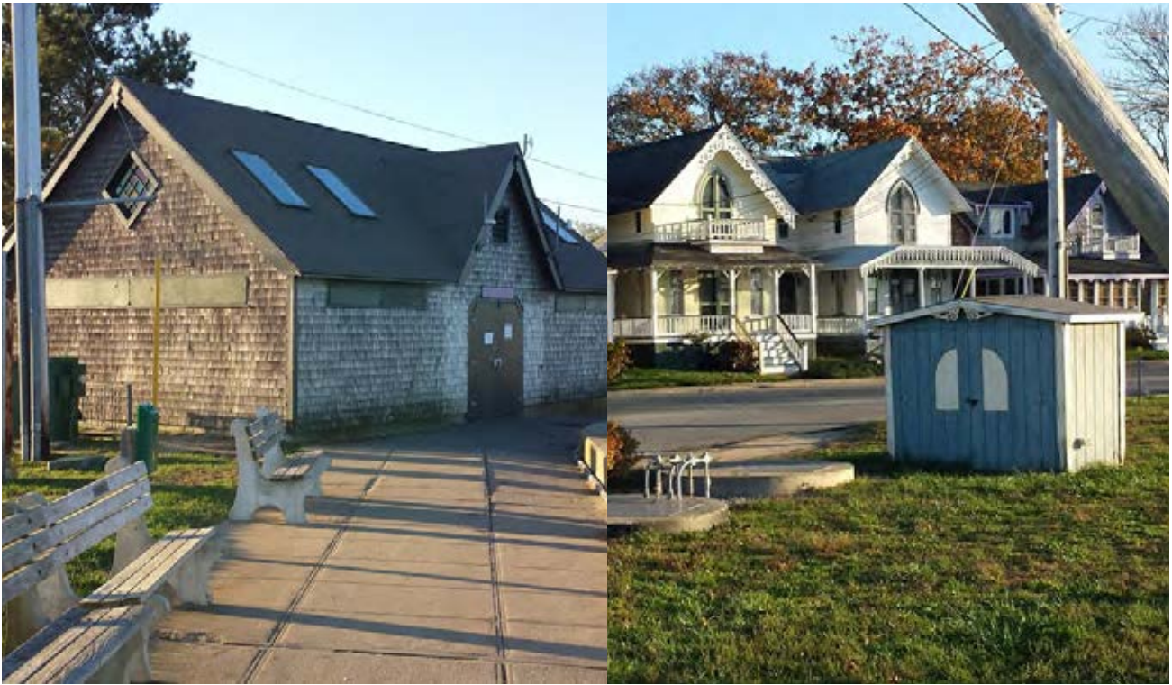
Electrical and sewer pump utilities along Lake Ave control important townwide infrastructure. These particular utilities are vulnerable to storm surge and flooding.
