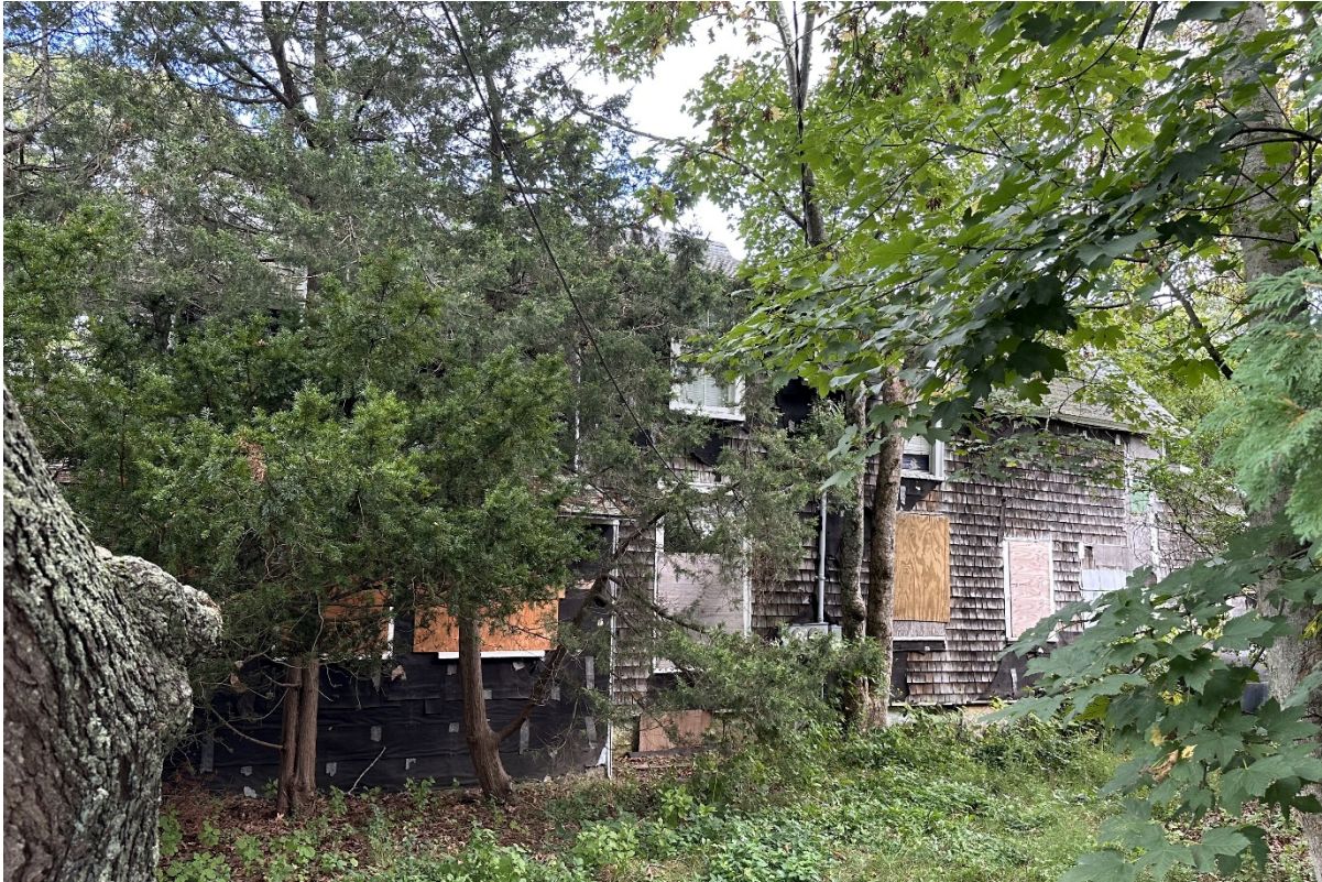
Photo 4. View of right side elevation from Circuit Avenue, looking east (September 2023).
