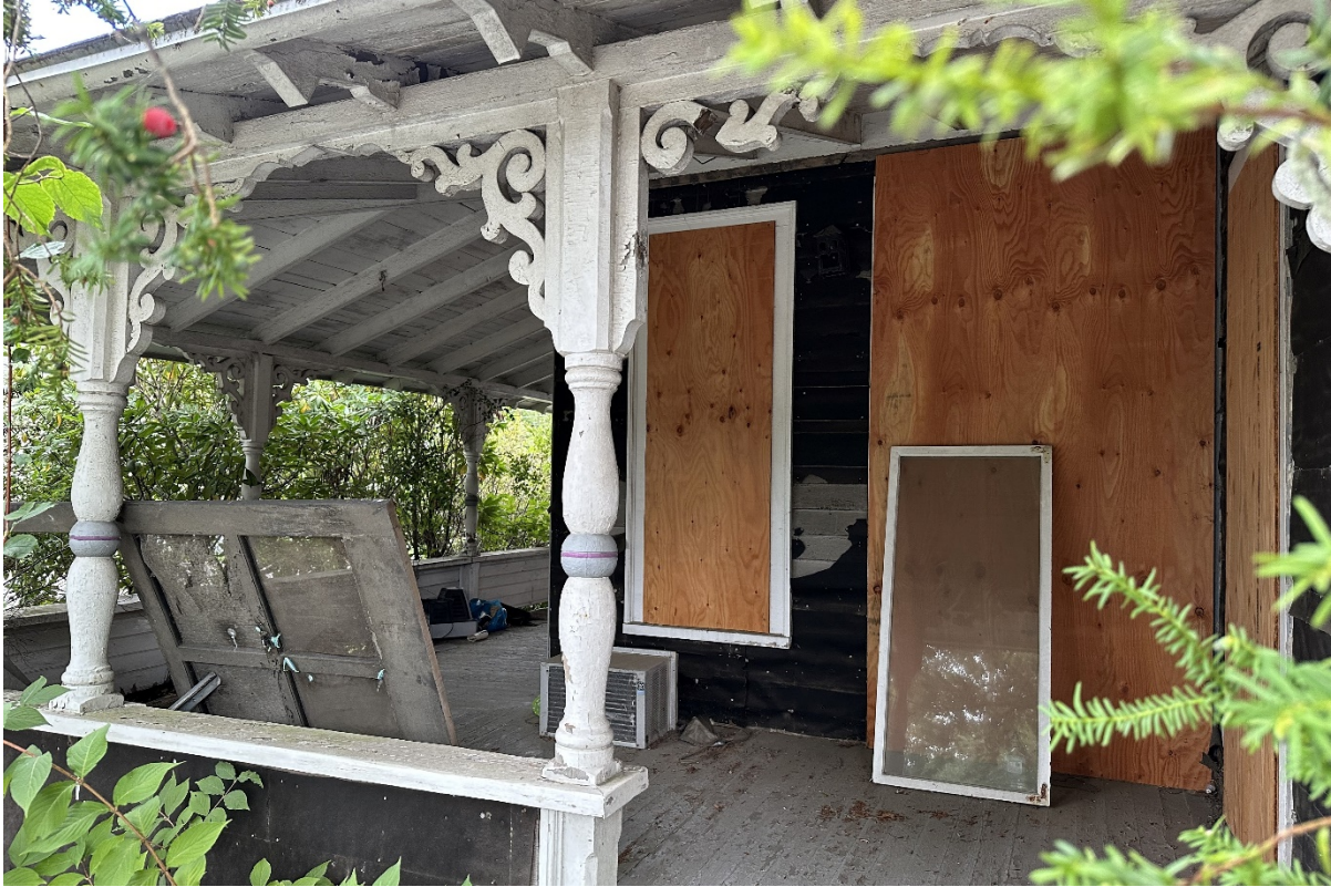
Photo 5. View of 3 Uncas Avenue front porch from Circuit Avenue, looking SE (September 2023).
