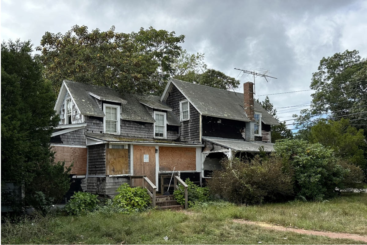
Photo 3. View of 3 Uncas Avenue from Uncas Avenue, looking west (September 2023).
