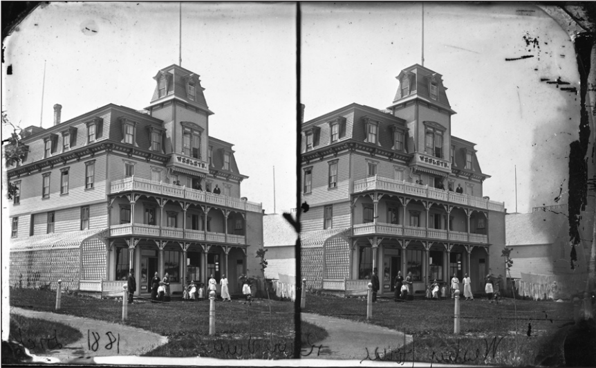
Fig. 13—The Lake Avenue façade of the hotel: Now the front, but originally—and when this picture was taken—the back of the building.
