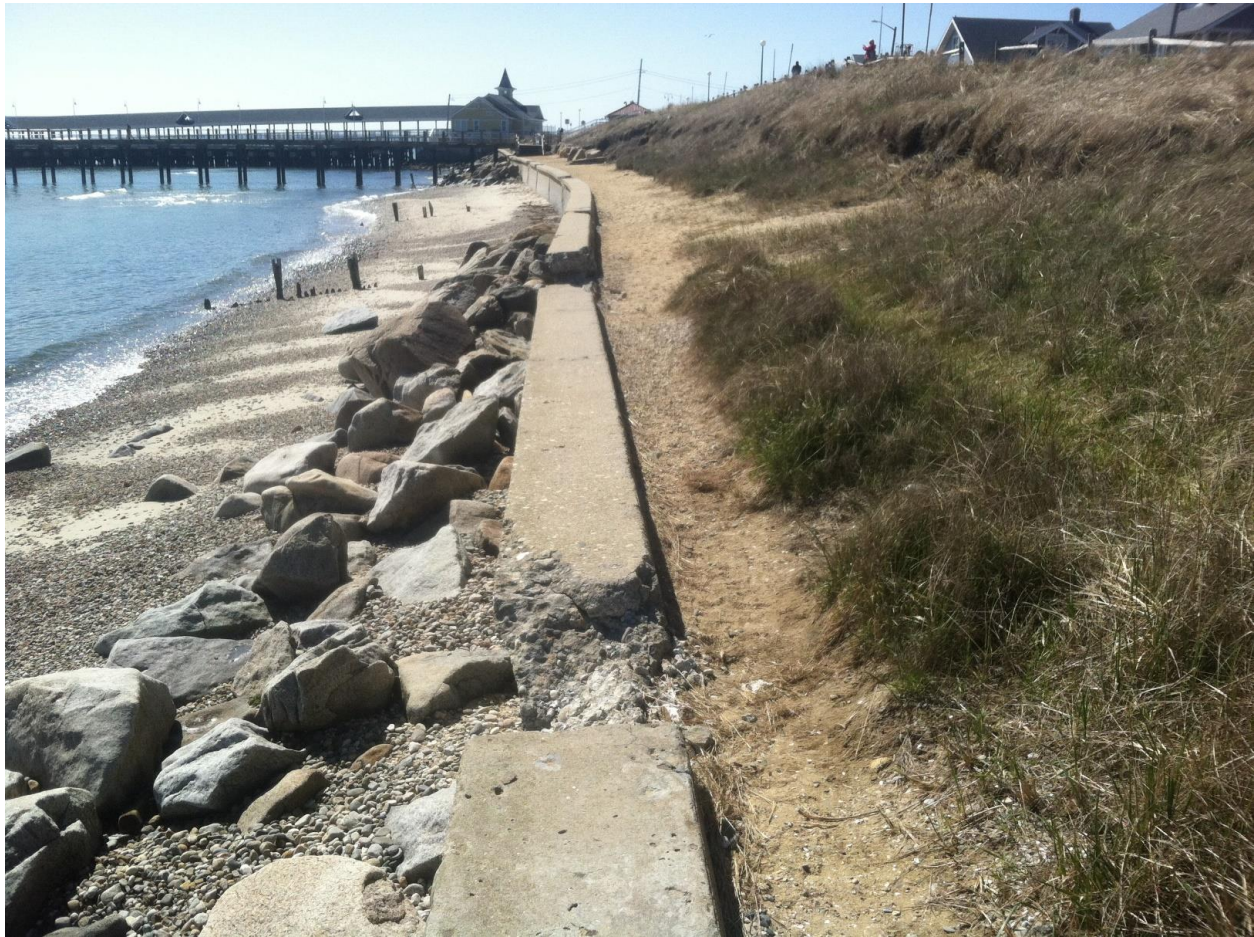
View of the North Bluff Seawall (2014)
