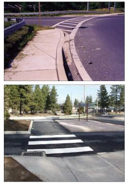
Place curb ramps in line with the pedestrian crossing to properly guide pedestrians across the approach. A curb ramp such as the one shown in the photo *should be avoided*, as it directs pedestrians into the path of vehicles traveling on the circulatory roadway instead of in the direction of the striped crossing.
