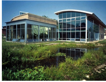
Wastewater Treatment, Oberlin College
