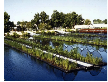
Industrial Waste Treatment, Tyson Food
