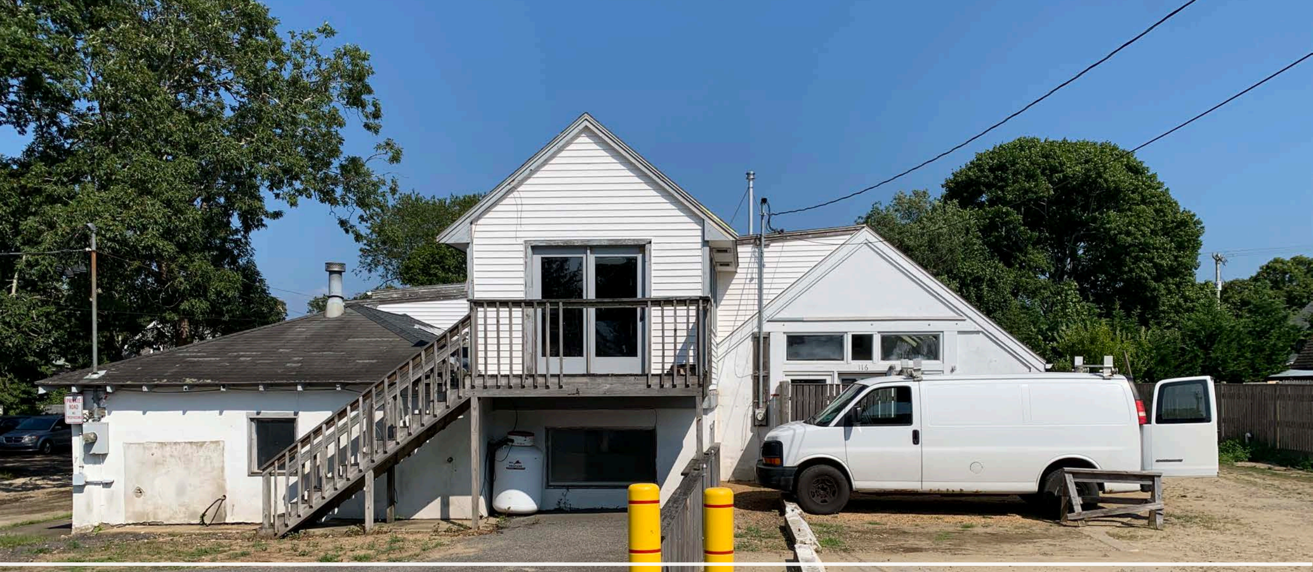
Western Side of Structure
