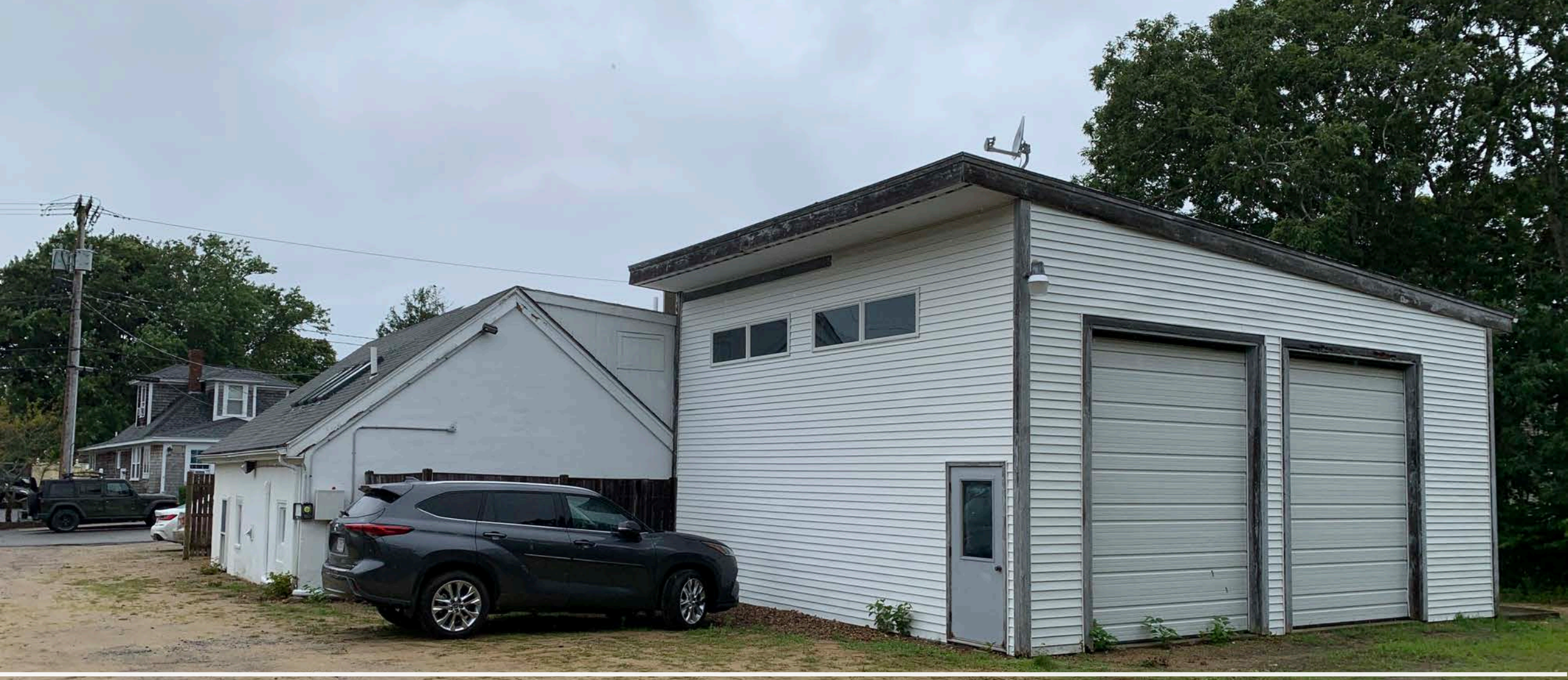
Eastern Side of Structure
