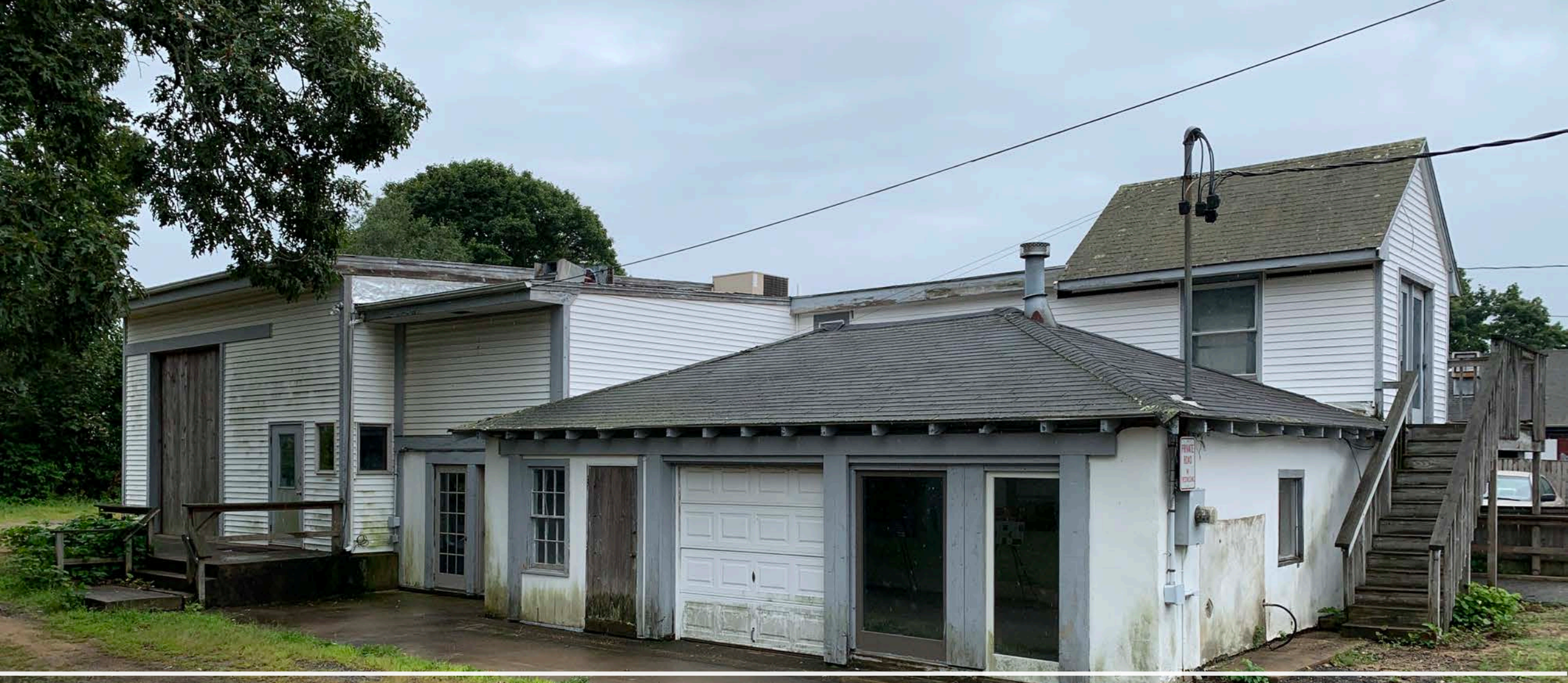
Northern Side of Structure
