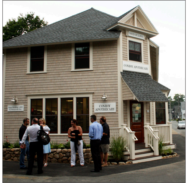
Noyes building in downtown Oak Bluffs, reinvented as a pharmacy and three affordable apartments. (Ivy Ashe/Vineyard Gazette)
