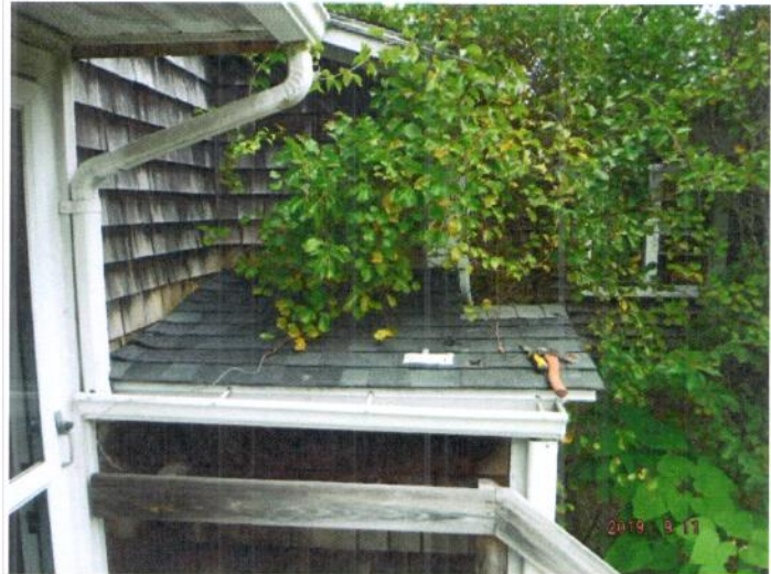
Samle 473-1 Shed roof Asphalt Shingle
