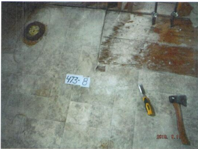
Sample 473-8 Middle bathroom flooring Sheet Vinyl
