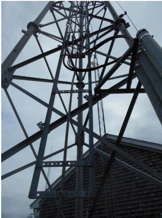
Photos of existing feed lines and feed line ladder on tower
