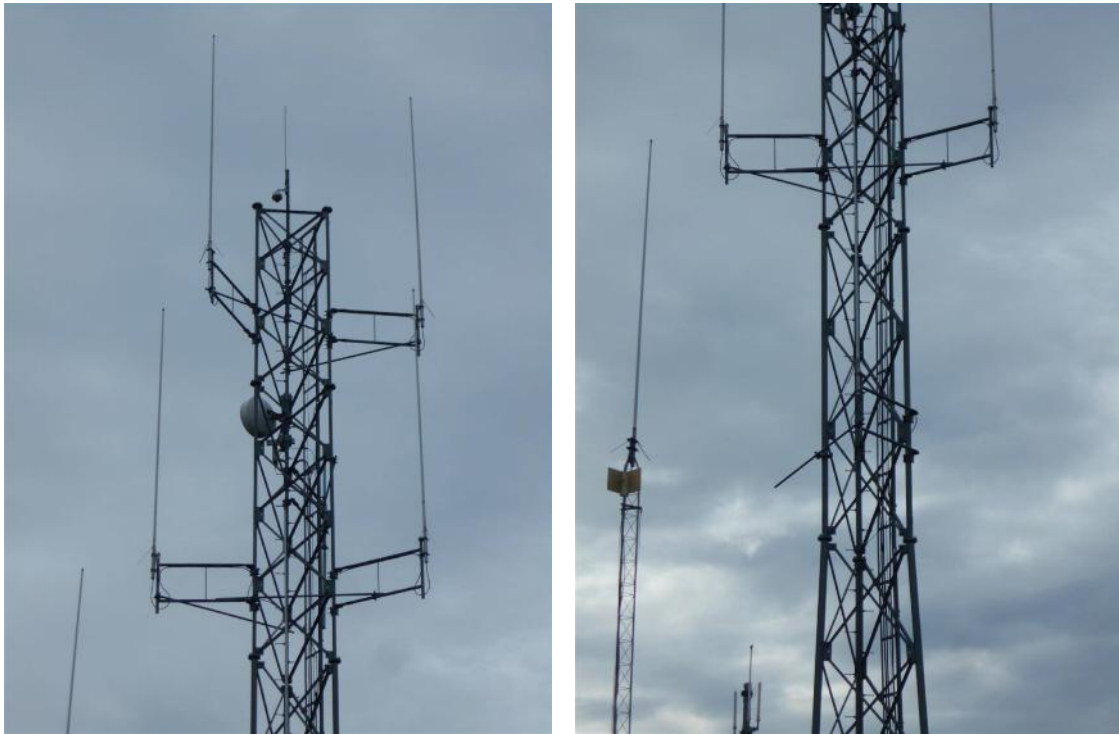
Photos of existing equipment on tower
