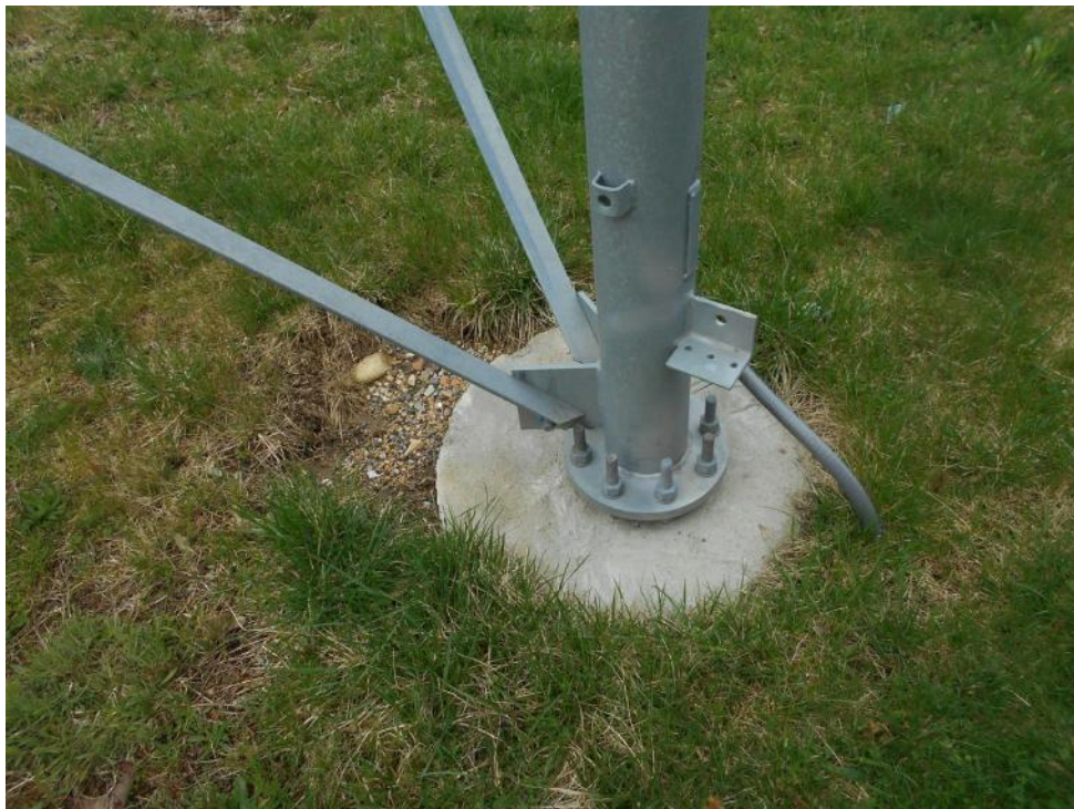
Photos of typical leg connections to foundation concrete
