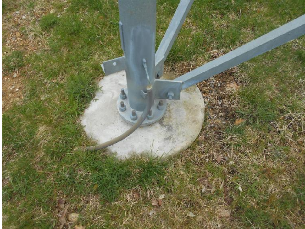
Photos of typical leg connections to foundation concrete
