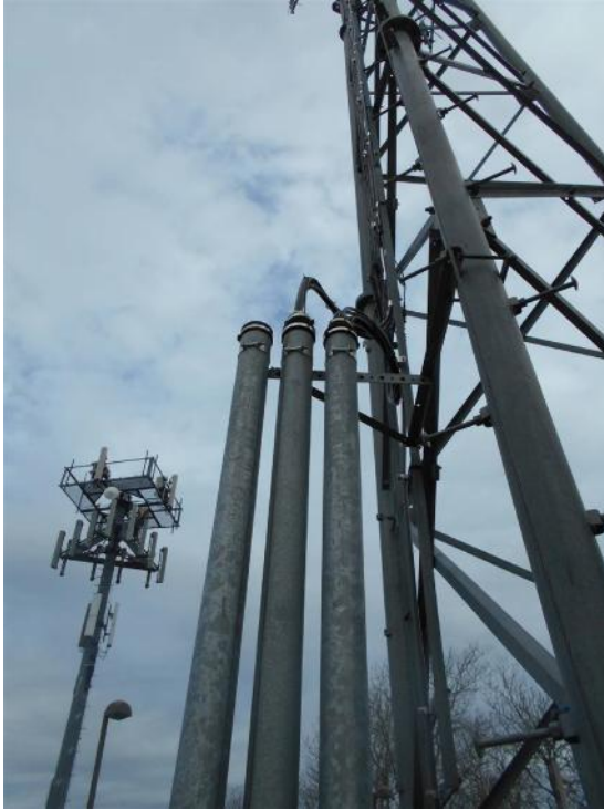
Additional photos of existing feed lines emerging from pipe conduit
