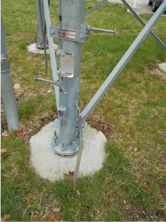
Photos of base of tower leg, and safety climb connection to tower leg
