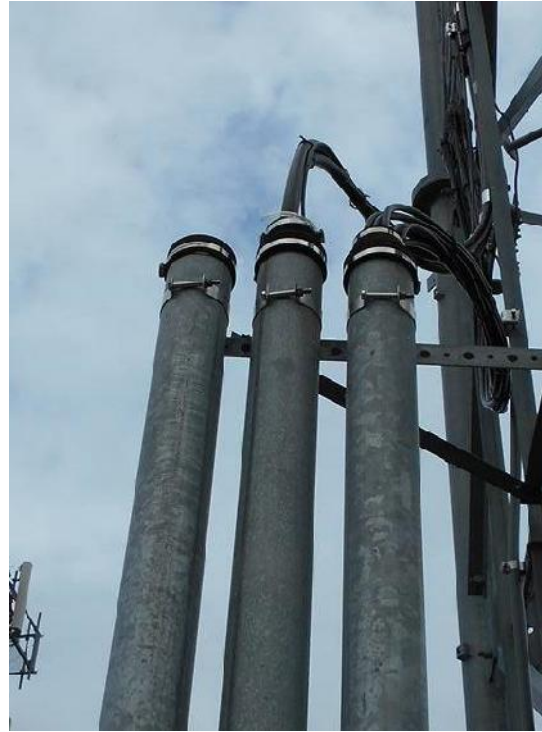
Additional photos of existing feed lines emerging from pipe conduit
