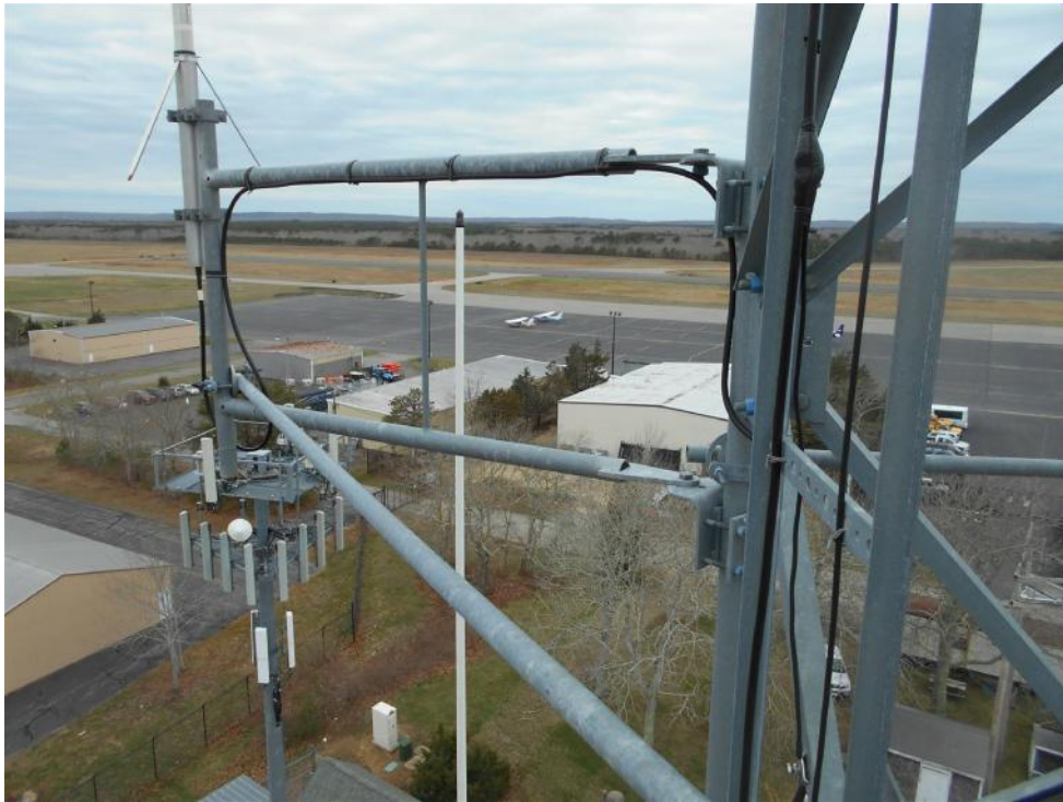
Photo of typical sidearm mount and stabilizer
