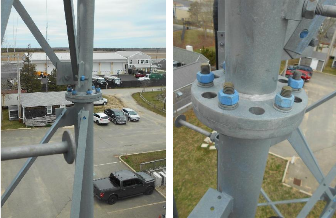
Photos of typical splice connection
