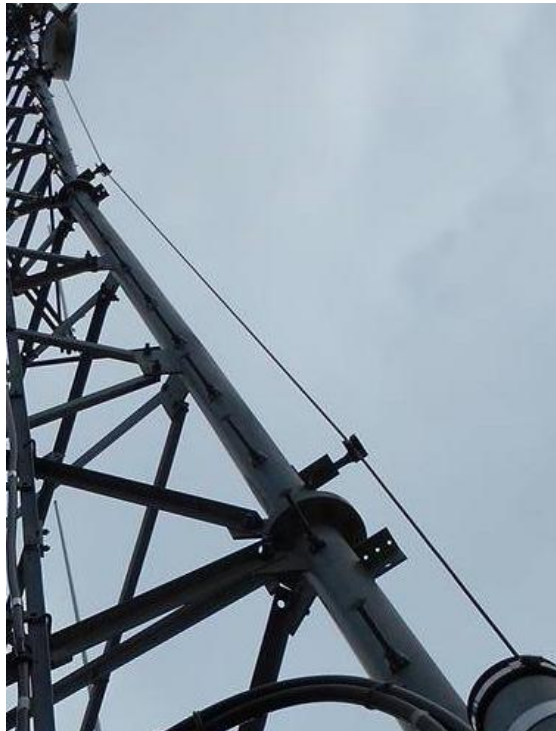
Photos of safety climb and climbing pegs on tower
