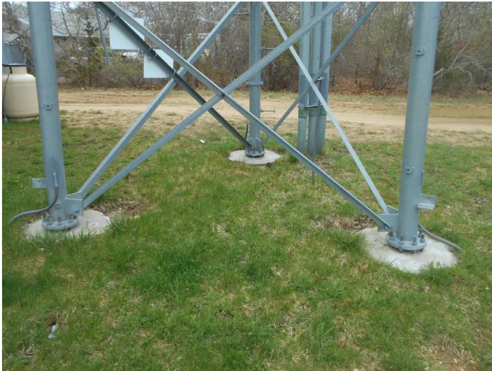
Photo of tower base, including anchor bolts and visible foundation concrete
