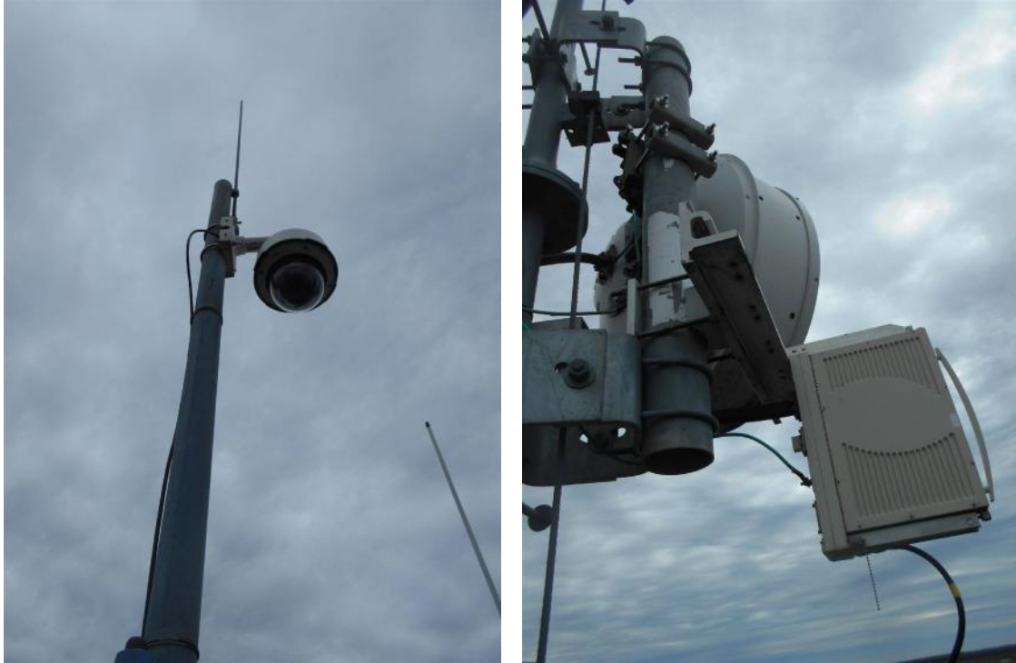
Photos of lightning rod and camera (left), and microwave dish with panel (right)
