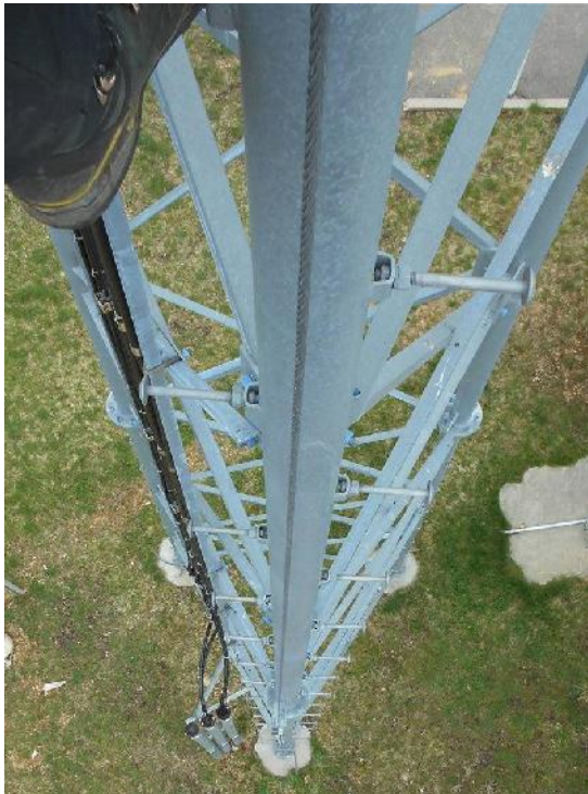
Photos of safety climb and climbing pegs on tower
