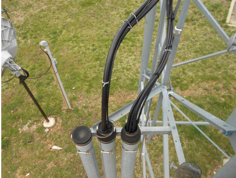
Photos of existing feed lines emerging from pipe conduit
