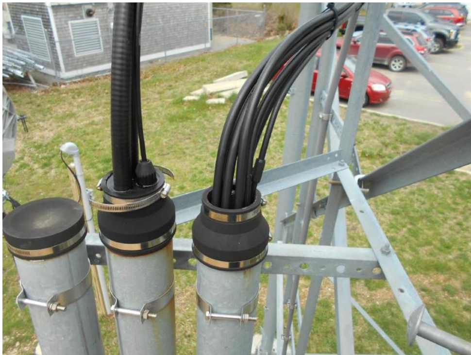
Photos of existing feed lines emerging from pipe conduit
