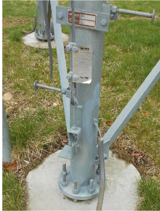
Photos of base of tower leg, and safety climb connection to tower leg
