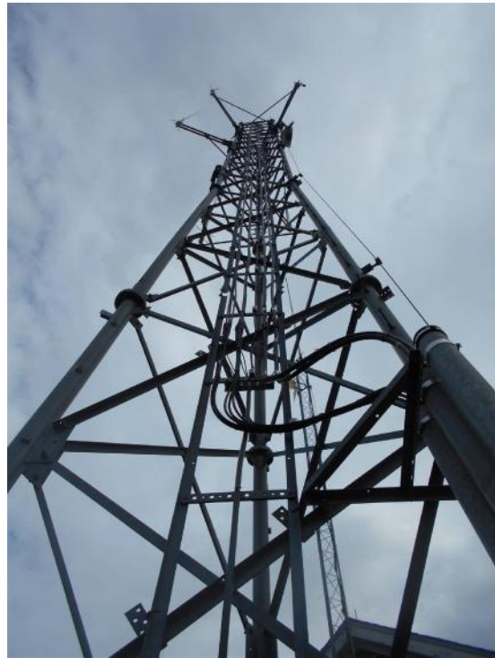
Photos of existing feed lines and feed line ladder on tower
