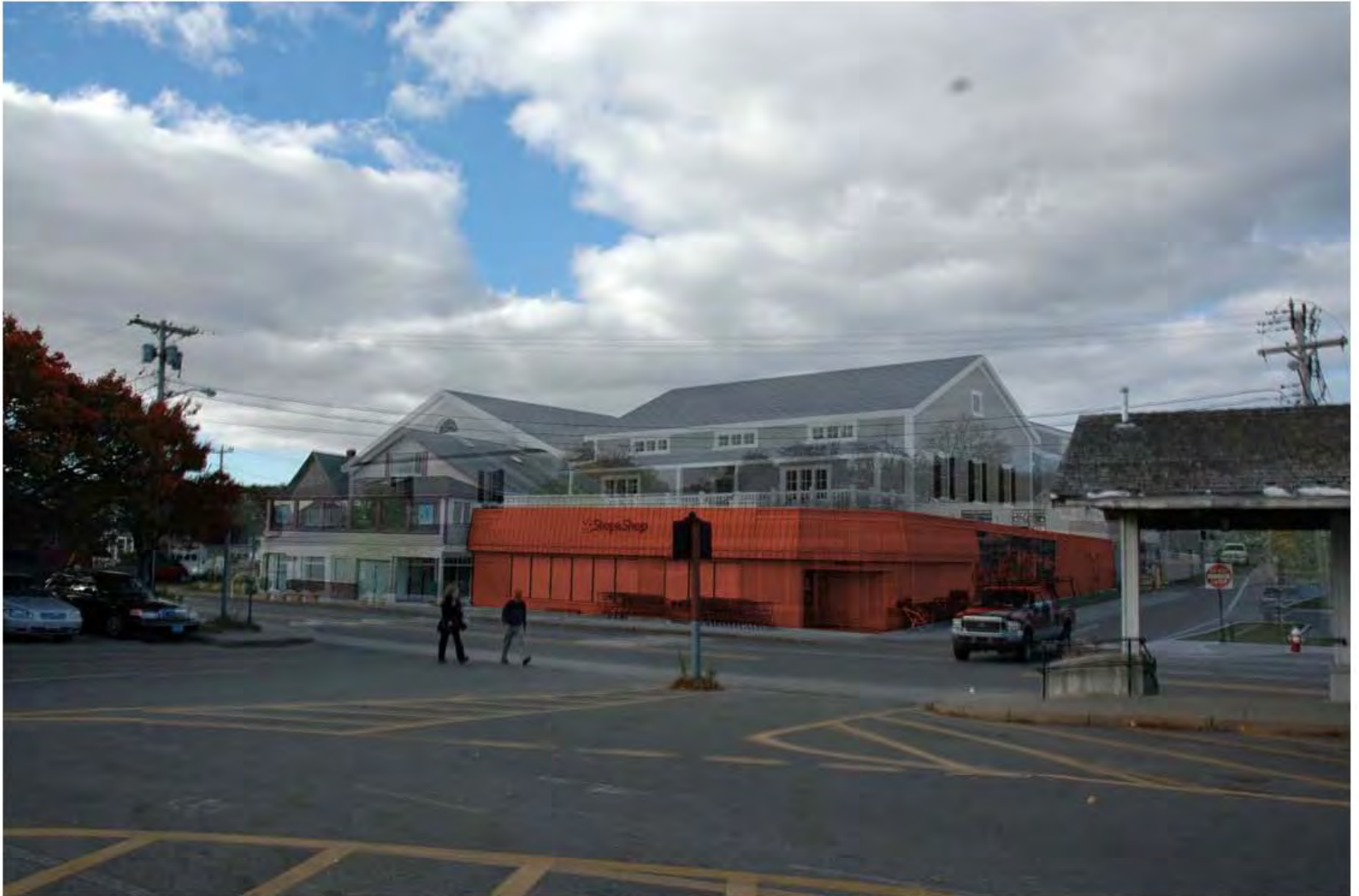
(NE Elevation-After) from SSA terminal vehicle standby area
