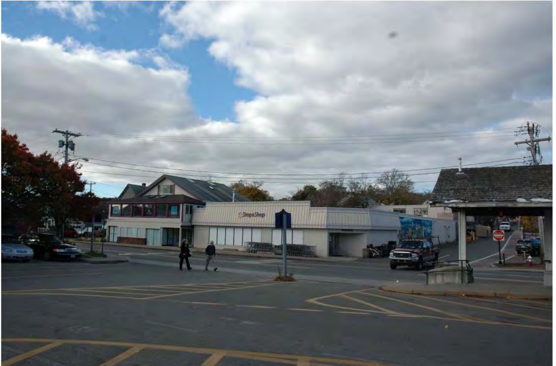
(NE Elevation-Before) from SSA terminal vehicle standby area
