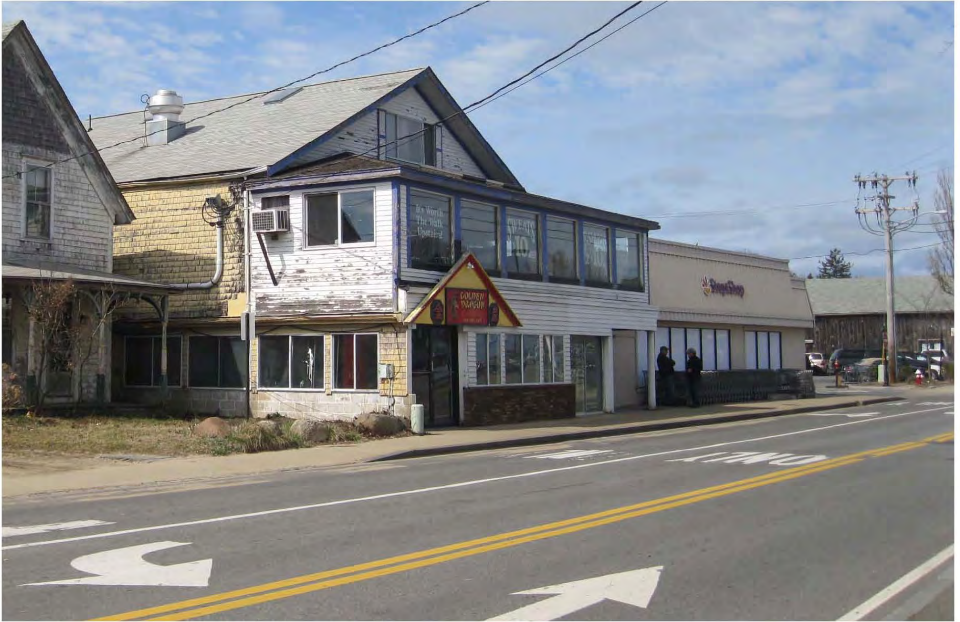
(SE elevation-Before) From Corner Five, Water St
