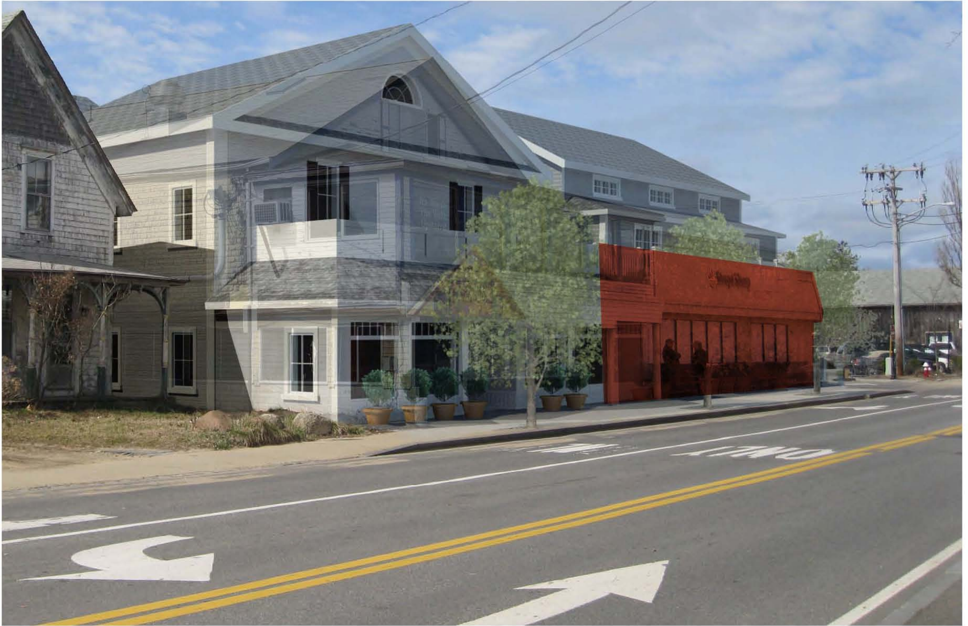
(SE elevation-After) From Corner Five, Water St
