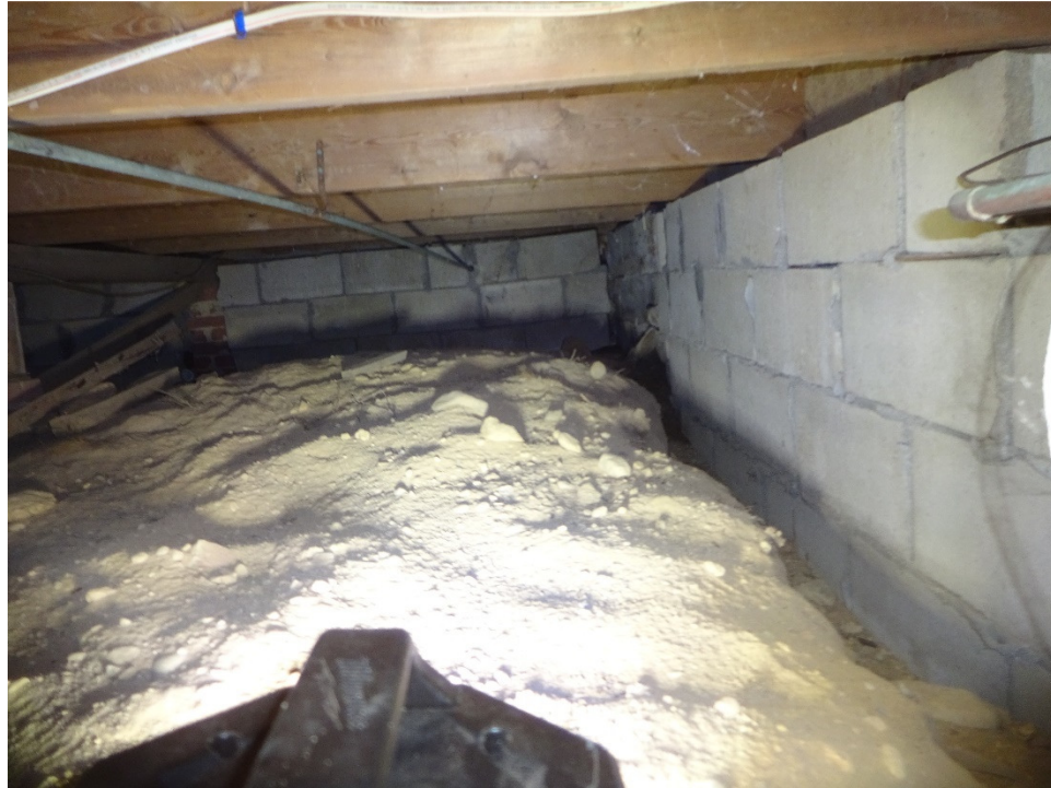
Figure 12: Non-Backfilled Perimeter Masonry Wall
