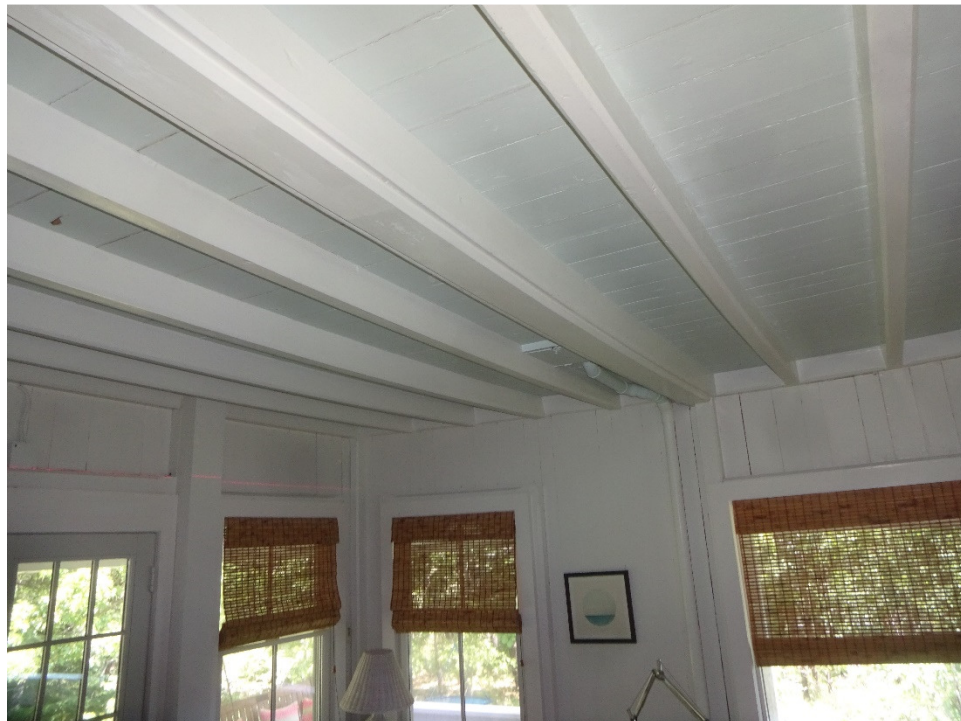
Figure 14: Second-Floor Framing Below Tower Structure
