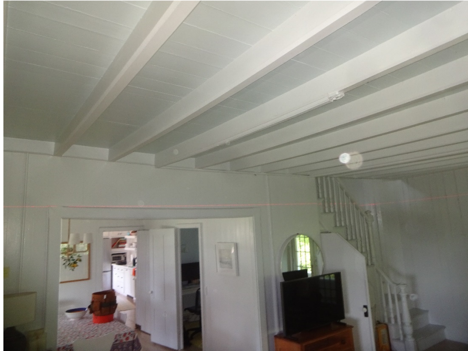
Figure 8: Second-Floor Framing Members over the Living Room
