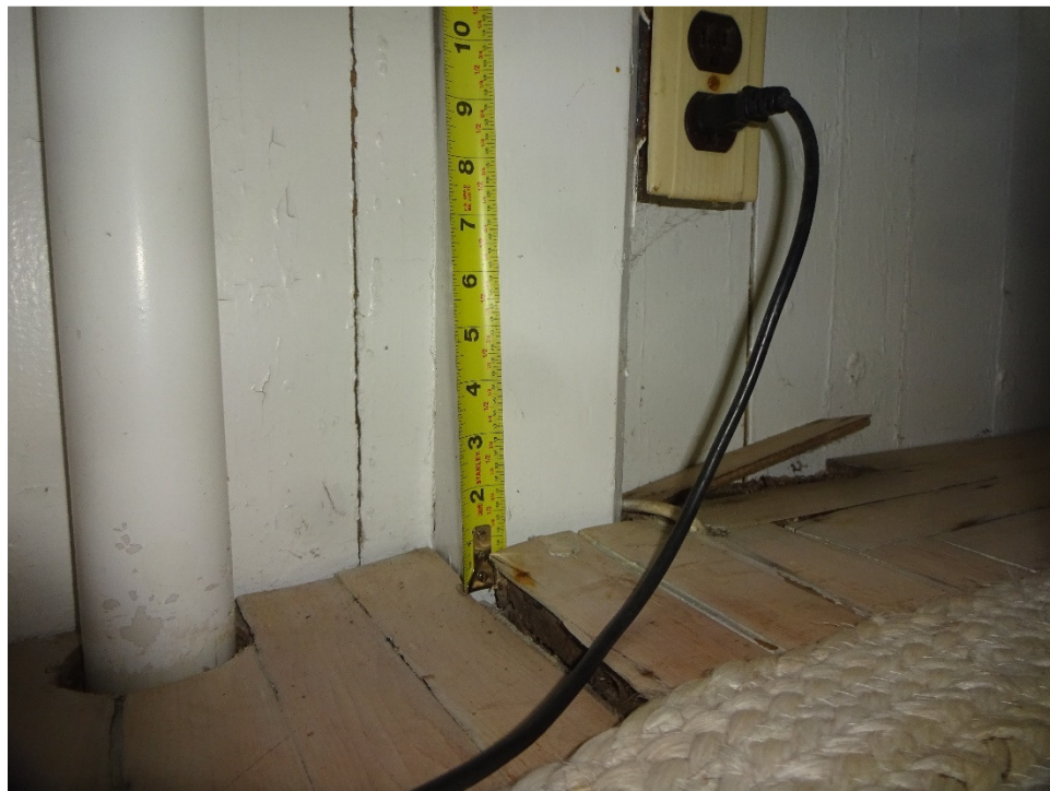
Figure 7: Step in First-Floor @ NE Corner of Main Structure
