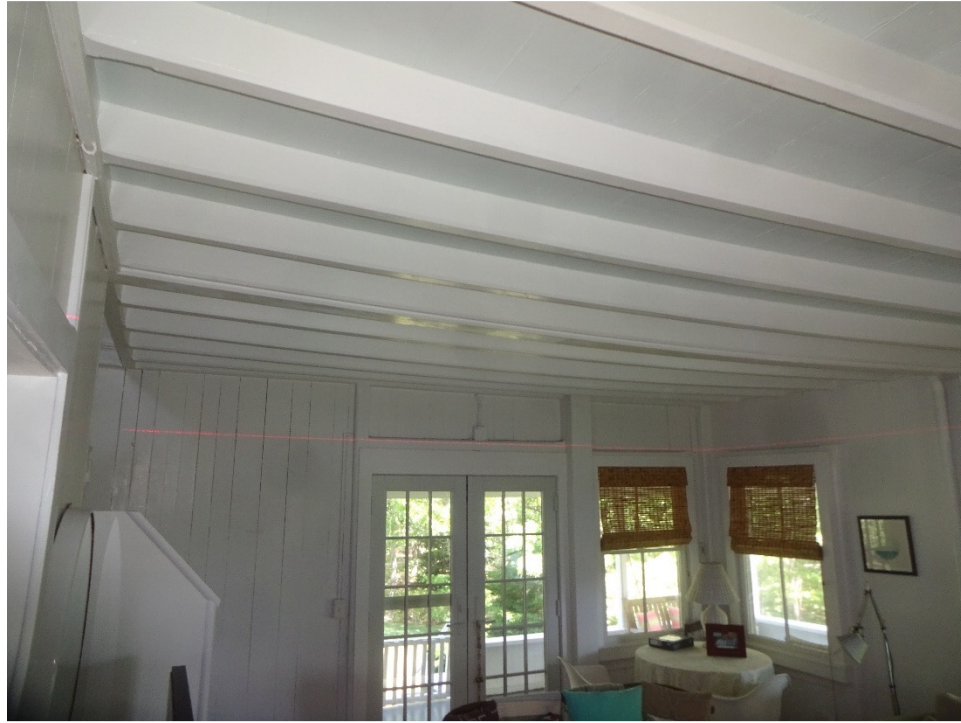
Figure 9: Northeast Corner Wall Framing
