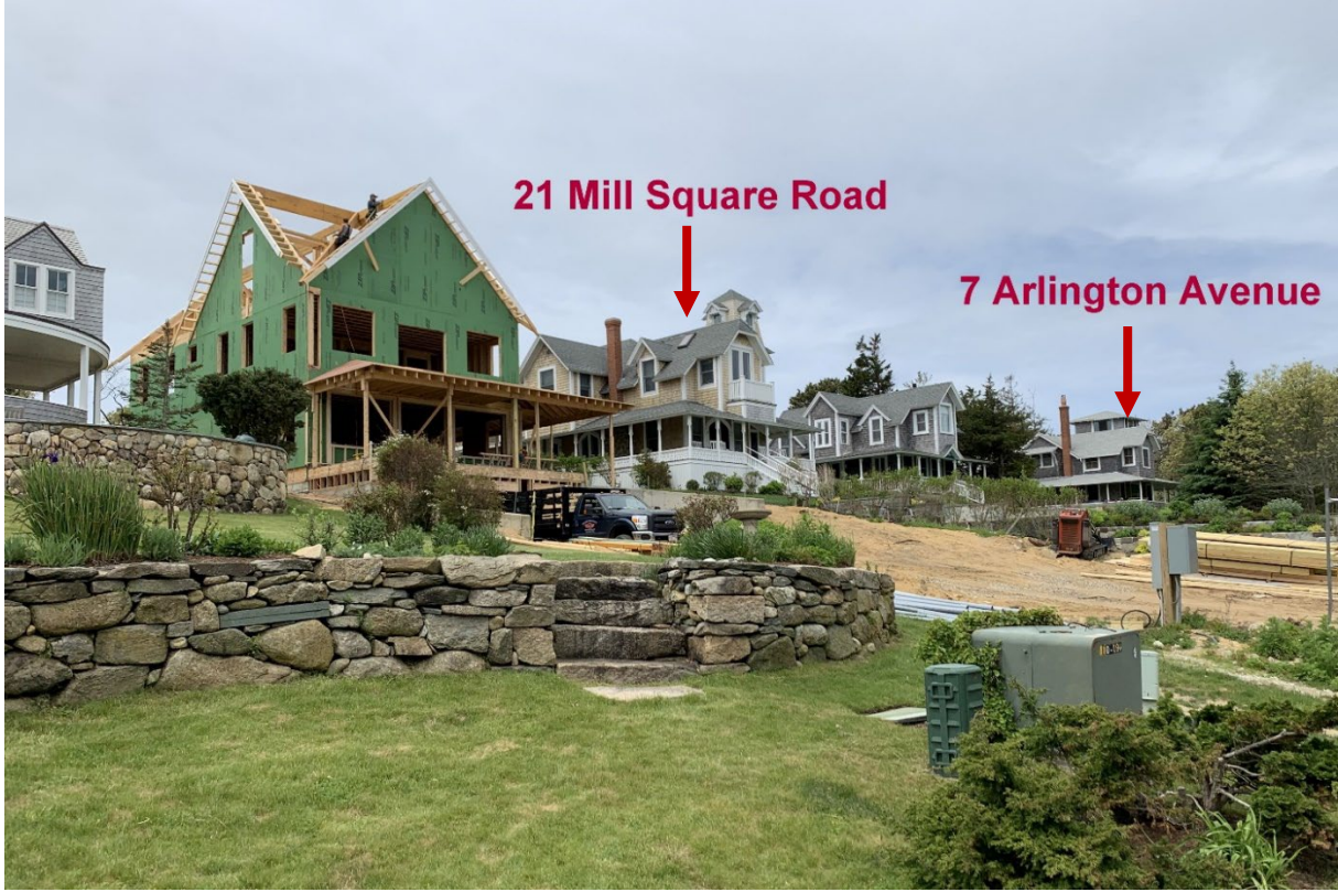
Photo 6. View looking north from East Chop Drive (annotated).
