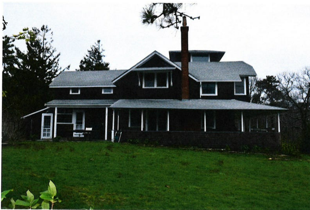
Photo 4. South elevation of 7 Arlington Avenue, view north.
