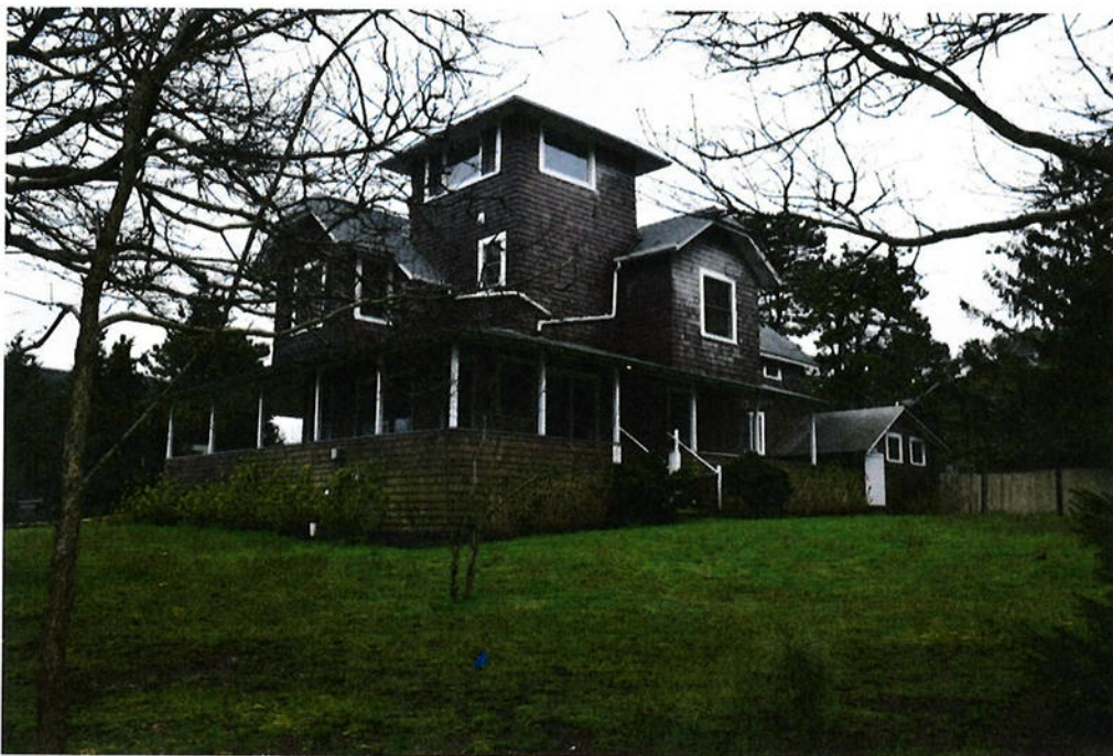
Photo 2. North and east elevations of 7 Arlington Avenue, view southwest.
