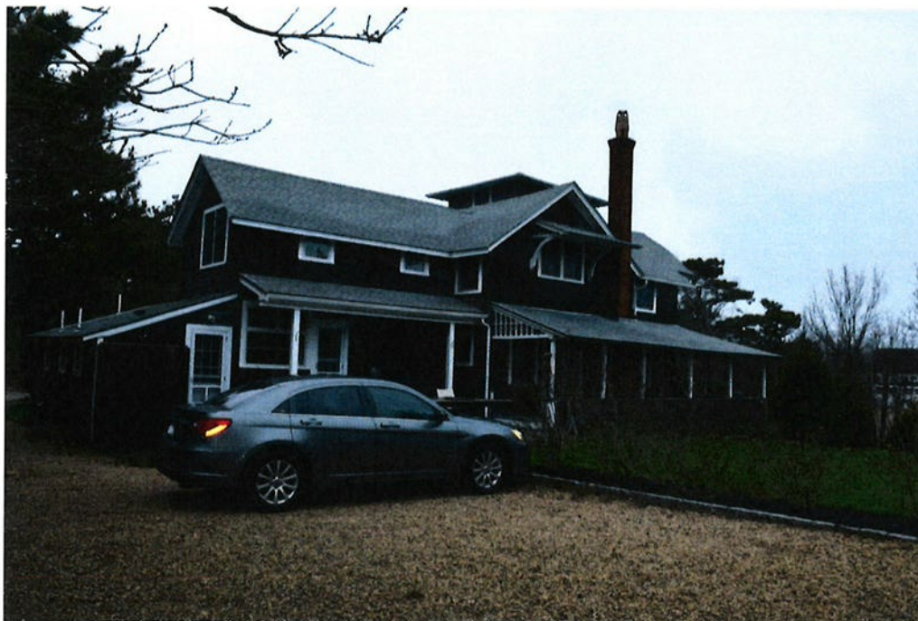
Photo 5. South and partial west elevations of 7 Arlington Avenue, view northeast.
