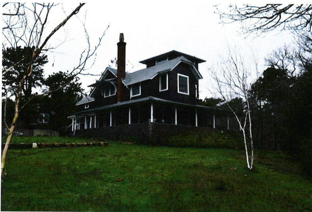
Photo 3. East and south elevations of 7 Arlington Avenue, view northwest.
