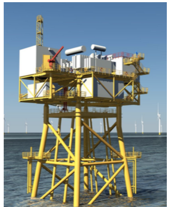
Rendering of an offshore substation (Deepwater Wind)
