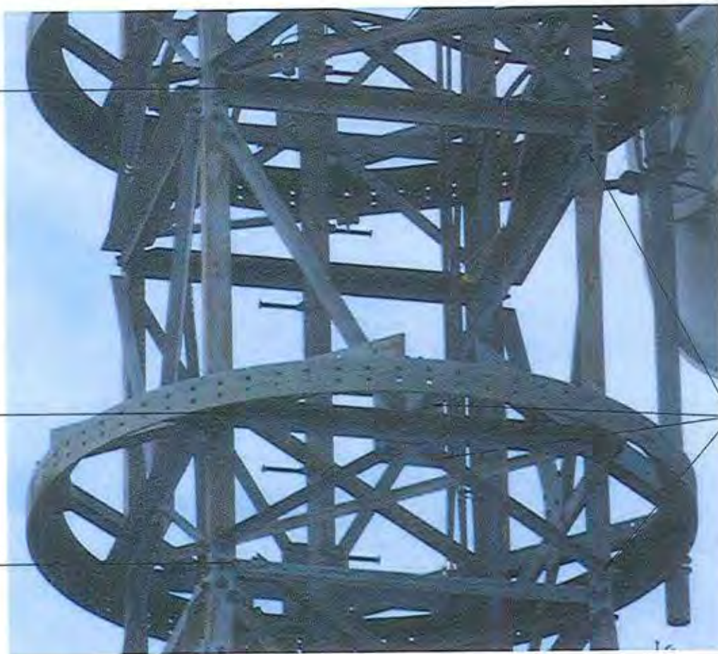
CP-02374-01 2x2x3/8" REPLACEMENT DIAGONAL 45'-4" TO 47'-5"
