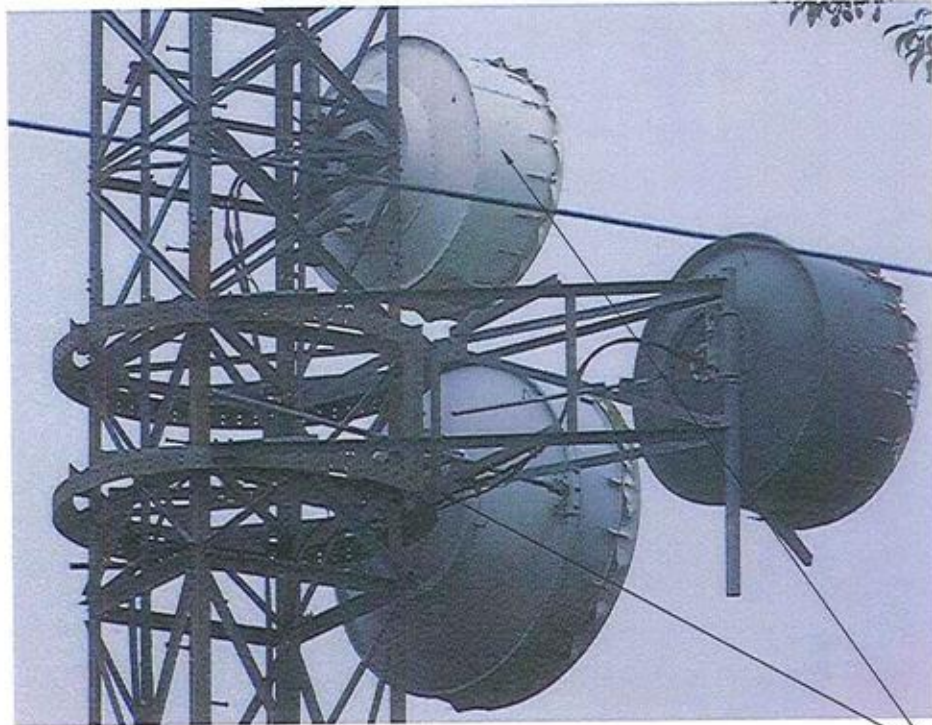
THE (3) DISHES AND MOUNTS FROM 55' TO 65' ARE TO REMAIN ACTIVE DURING CONSTRUCTION. THE ANGLE-X FROM 45'-4" TO 65'-2" IS TO BE INSTALLED LAST SO THESE DISHES CAN REMAIN ACTIVE. ONCE ALL OF THE REINFORCEMENTS AND TOWER EXTENSION HAVE BEEN INSTALLED RE-LOCATE THESE (3) DISHES AND MOUNTS TO THE TOWER EXTENSION. AFTER THESE DISHES AND MOUNTS HAVE BEEN RE-LOCATED TO THE TOWER EXTENSION THE ANGLE-X FROM 45'-4" TO 65'-2" IS TO BE INSTALLED.
