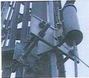
EXISTING SAFETY CLIMB TOP TERMINATION AT 33' TO BE REMOVED PRIOR TO ANGLE-X INSTALLATION.
