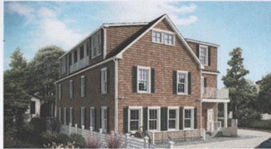
REAR AS BUILT VIEW
