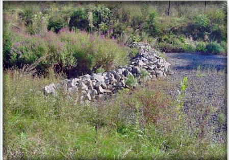
**Description:** A sediment forebay is a post-construction practice consisting of an excavated pit, bermed area, or cast structure combined with a weir, designed to slow incoming stormwater runoff and facilitating the gravity separation of suspended solids. This practice is different from a sediment trap used as a construction period BMP.
