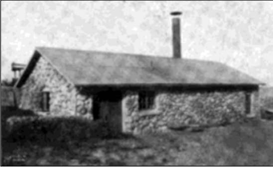
Luxemoor's Powerhouse. General Electric Review (GE's company journal) wrote an article about this outbuilding titled "A Model Small Isolated Plant." It begins: "Dreamy, picturesque Vineyard Haven! – probably the last place one would naturally expect to find an installation of man's latest and greatest development in the steam engineering line – the Curtis steam turbine."
