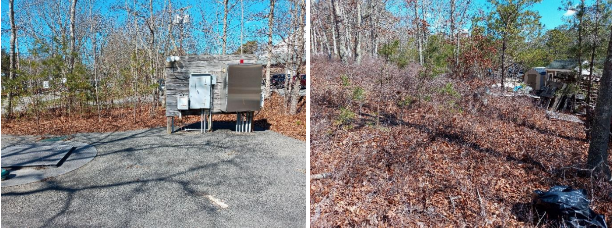
Photo 4. Existing sewer pump station and access drive in southwestern corner of site (left) and encroachment of structures and materials along southeastern property line (right).
