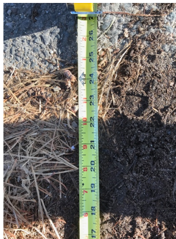
Photo #5: Detail of obscured road measurement
