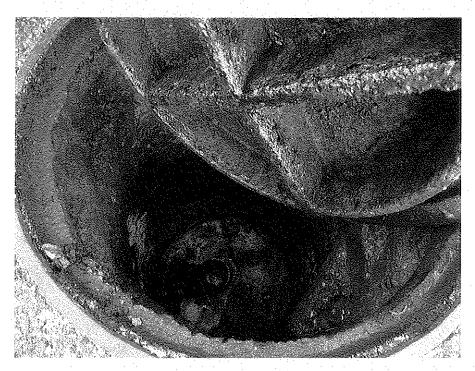
**12.)** Interior view of the second of the two covers for the grease separator system that is located behind and to the west of the Subject Property's building's rear.
