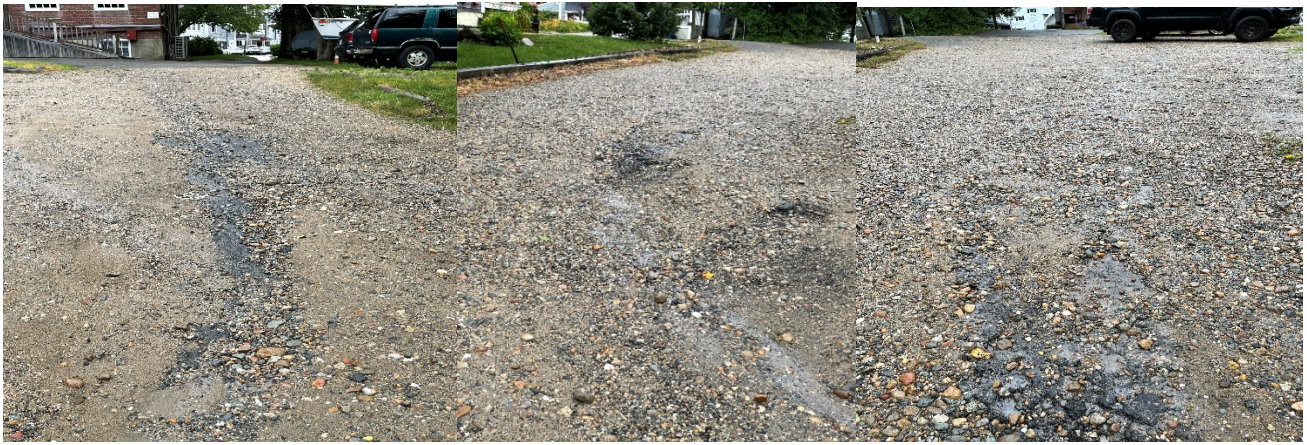
Parking area erosion caused by stormwater run-off.
