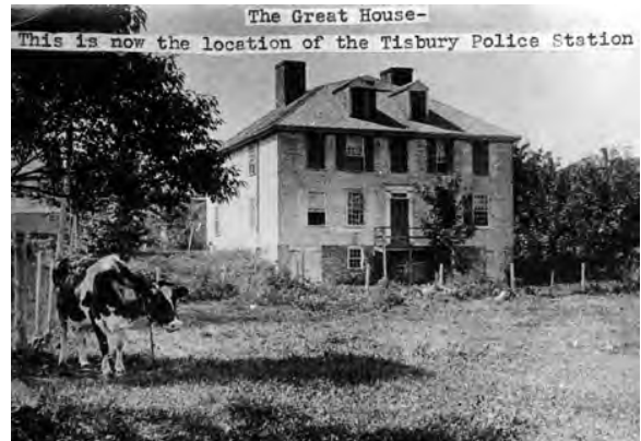
Great House, Water Street. Moved to West Chop in the mid twentieth century
