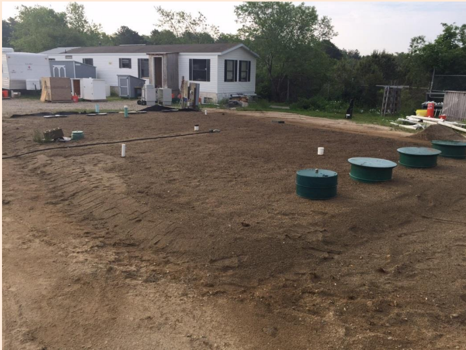
Final grade over soil treatment area
