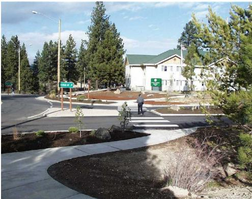
At a single lane roundabout, pedestrian crossings should be placed one vehicle length away from the entrance line as shown in the photo at left.
