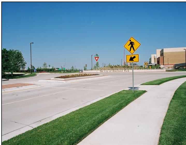
Landscaped planter strips set back the sidewalk from the adjacent roadway. This helps to define the sidewalk area and discourage pedestrians from crossing the roadway at locations other than the striped and/or signed crossing.
