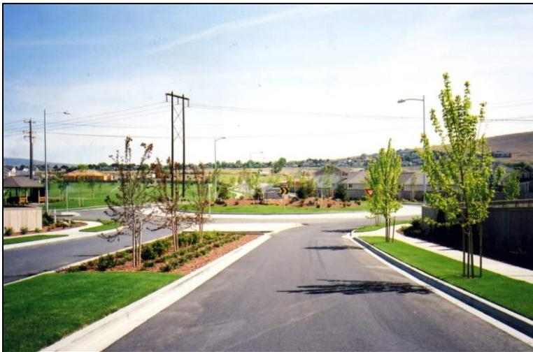
Landscaping within the splitter islands and along the outer edge of the approach can help create a funneling effect to help decrease speeds prior to the roundabout.
